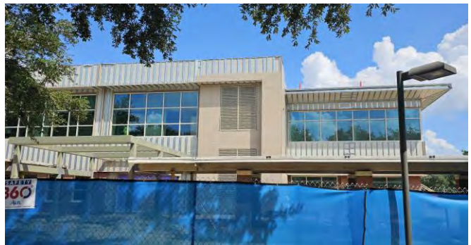
West side of building
