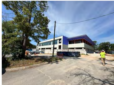
From walkthrough: Main entrance from parking lot (camera facing west)
