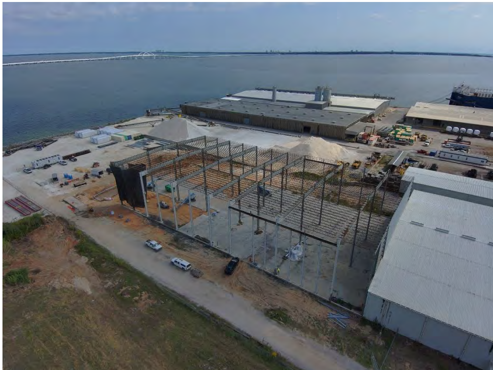
Aerial view of site on 10/15/24
