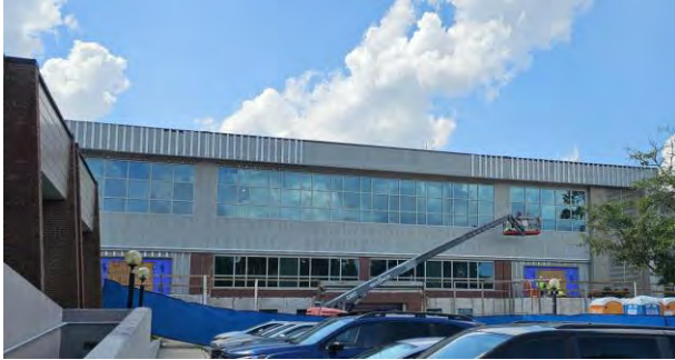
East side of building
