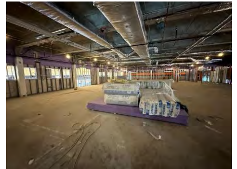
From walkthrough: Large classroom/lab space in center of building
