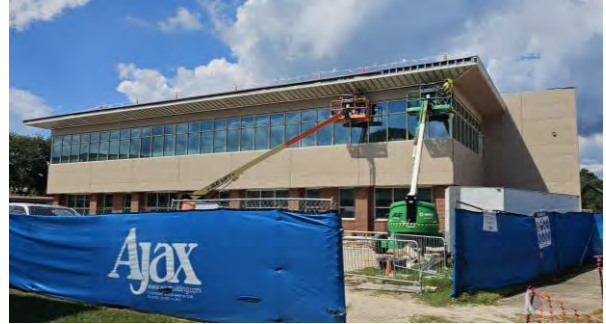
South side of building
