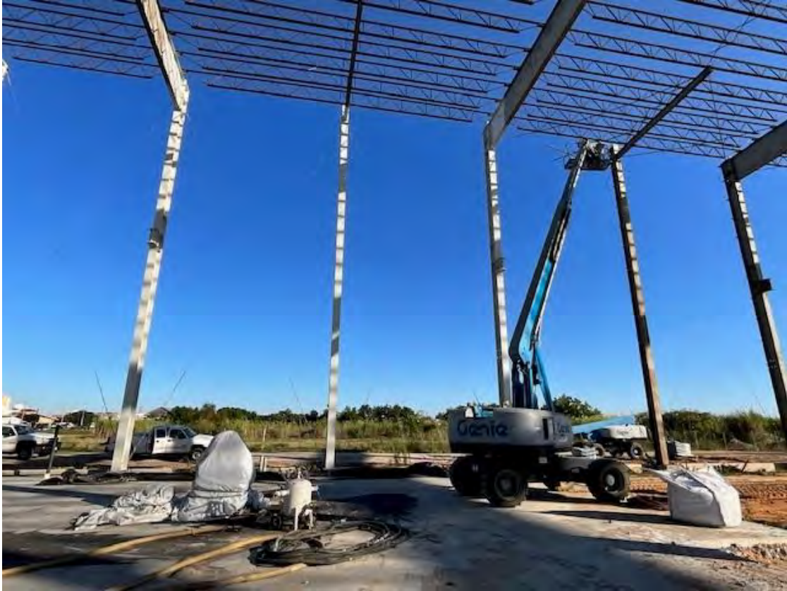
Existing steel beams being refurbished
