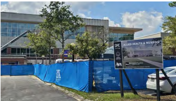
East side of building
